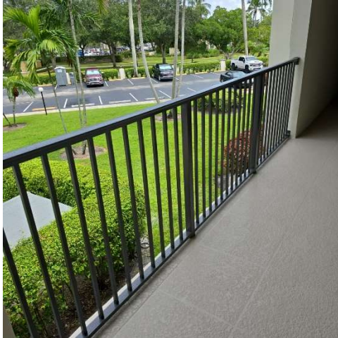
PHOTO-19 Typical Catwalk Guardrail
