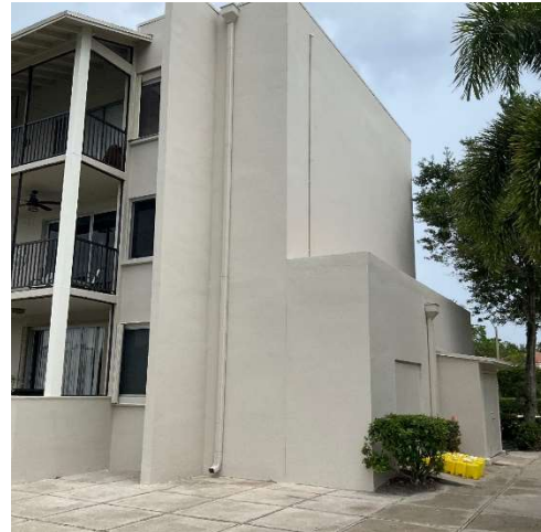
PHOTO-04 Building Exterior
