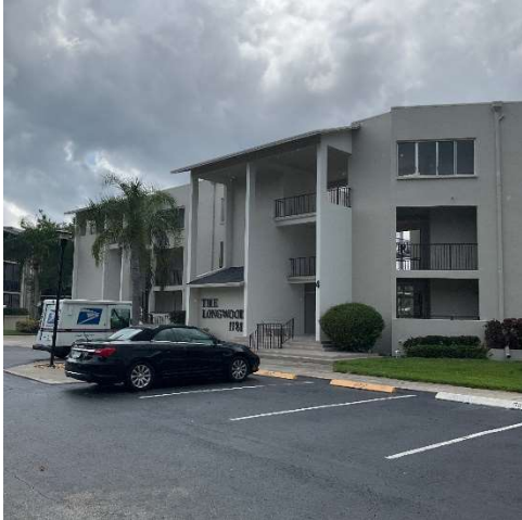
PHOTO-01 Building Exterior
