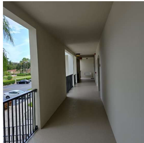
PHOTO-18 Typical Catwalk
