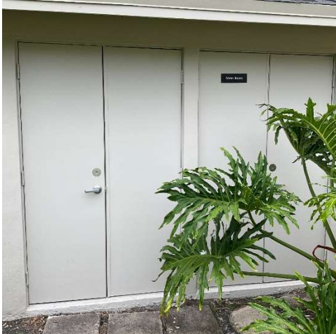
PHOTO-25 Typical Exterior Door
