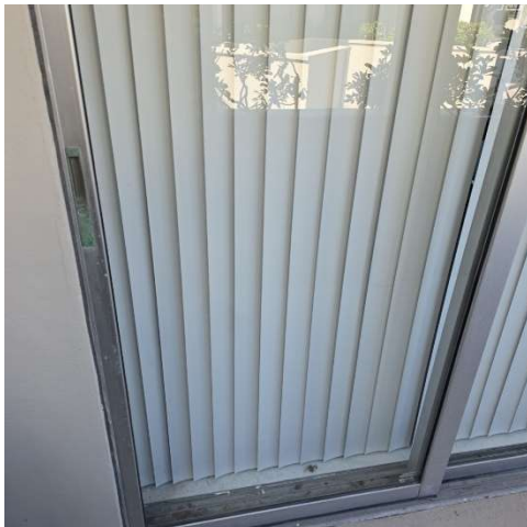
PHOTO-23 Typical Unit Sliding Glass Door
