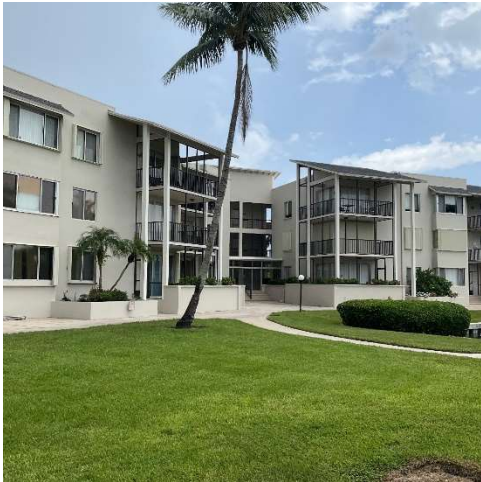
PHOTO-03 Building Exterior
