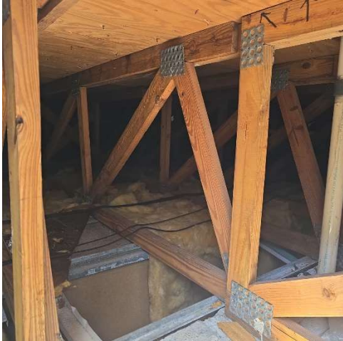
PHOTO-07 Roof Structure
