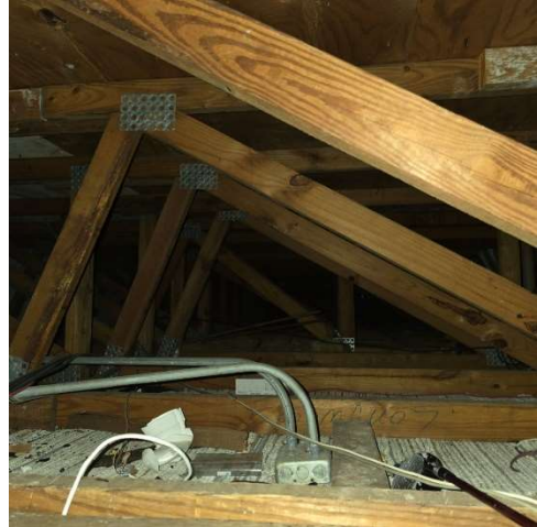
PHOTO-08 Roof Structure
