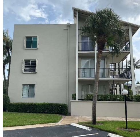
PHOTO-02 Building Exterior
