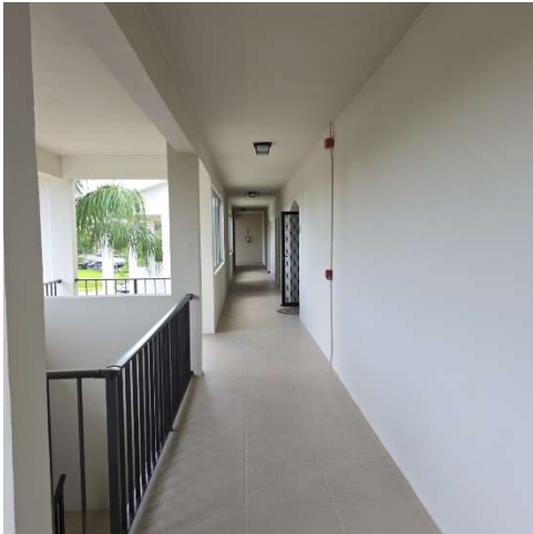
PHOTO-15 Typical Catwalk
