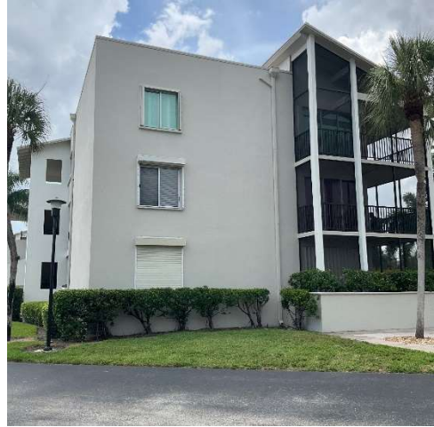
PHOTO-02 Building Exterior
