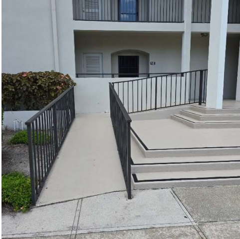
PHOTO-19 Entry Ramp
