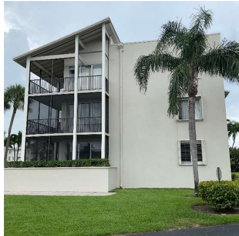
PHOTO-04 Building Exterior
