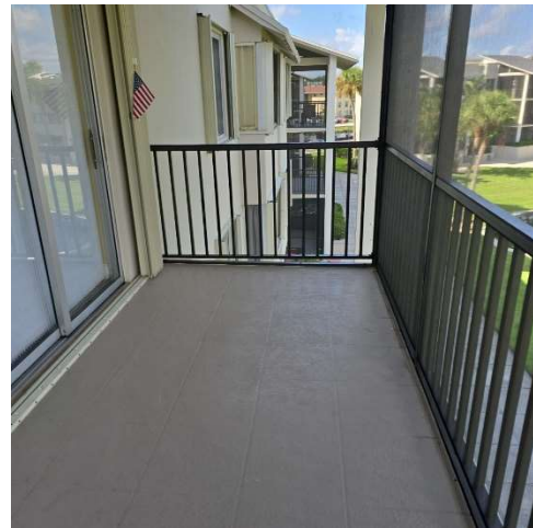
PHOTO-18 Typical Unit Balcony
