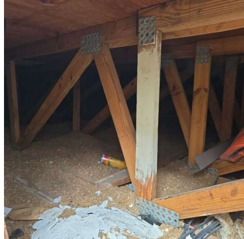
PHOTO-08 Roof Structure
