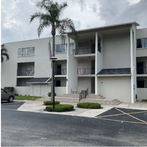
PHOTO-01 Building Exterior
