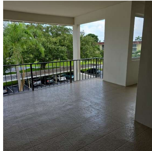
PHOTO-16 Typical Catwalk Guardrails
