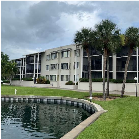
PHOTO-03 Building Exterior
