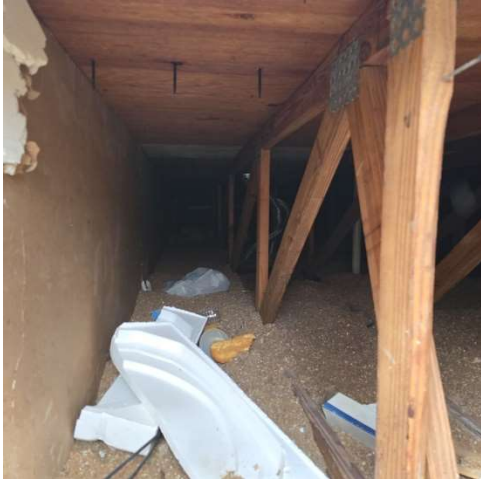
PHOTO-07 Roof Structure
