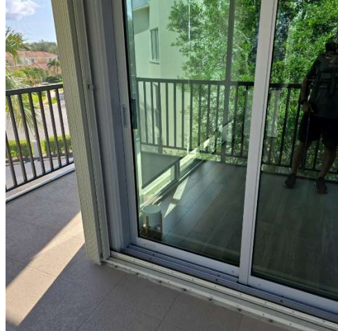
PHOTO-20 Typical Unit Sliding Glass Doors
