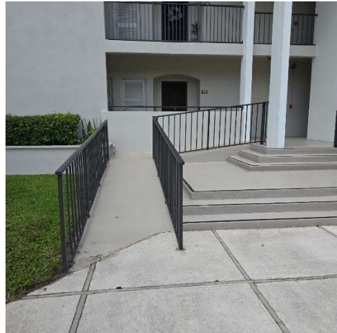
PHOTO-22 Entry Ramp
