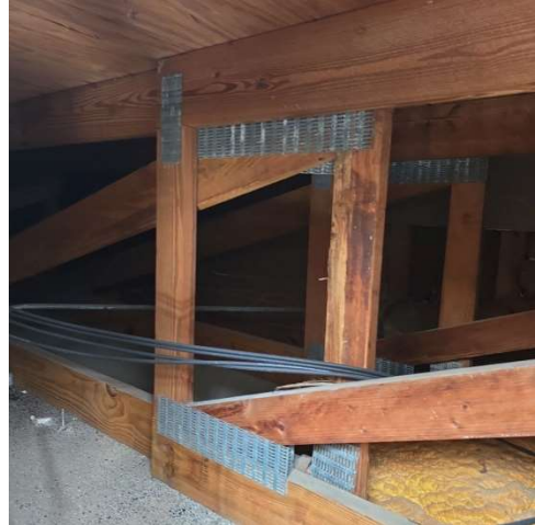
PHOTO-08 Roof Structure
