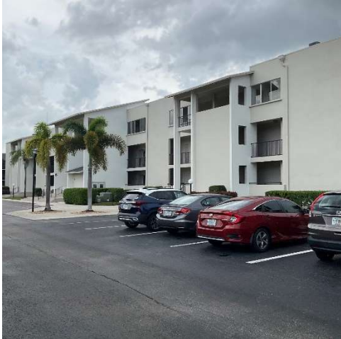
PHOTO-01 Building Exterior
