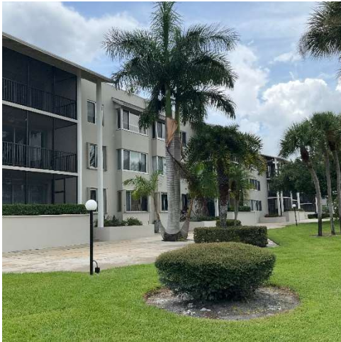
PHOTO-03 Building Exterior
