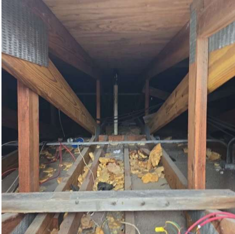
PHOTO-07 Roof Structure
