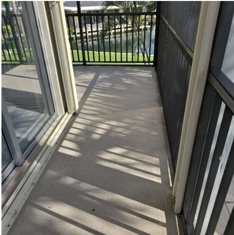
PHOTO-21 Typical Unit Balcony
