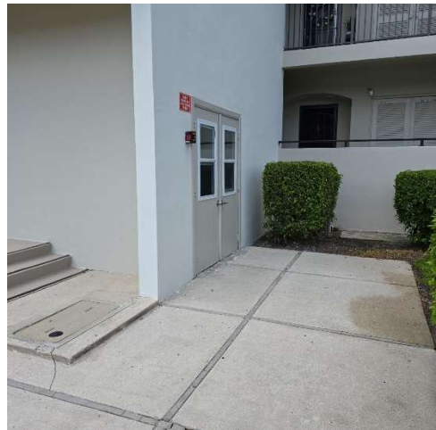
PHOTO-24 Typical Exterior Doors
