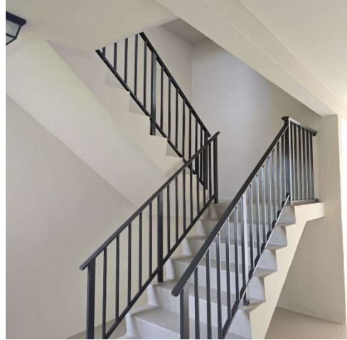
PHOTO-20 Typical Staircase
