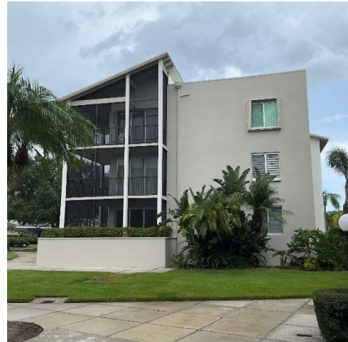
PHOTO-04 Building Exterior
