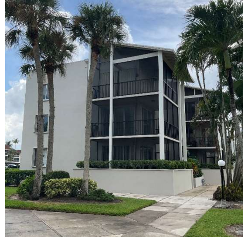
PHOTO-02 Building Exterior
