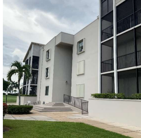
PHOTO-02 Building Exterior
