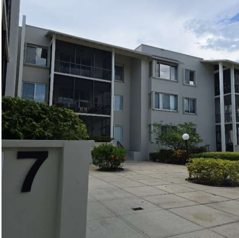
PHOTO-01 Building Exterior
