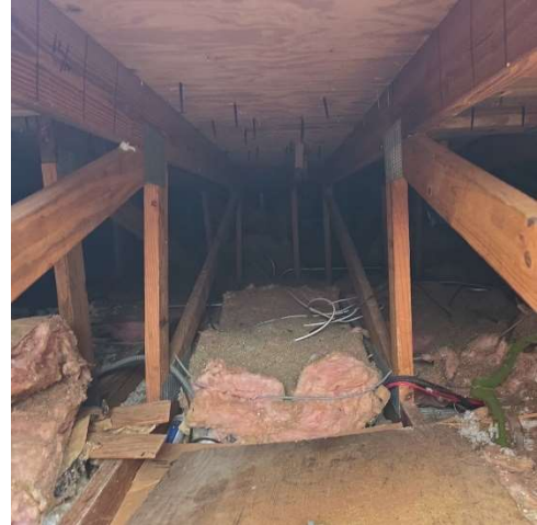
PHOTO-08 Roof Structure
