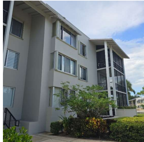
PHOTO-04 Building Exterior
