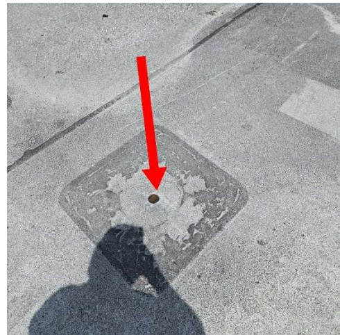
PHOTO-10 Typical Roof Drain Missing Dome
