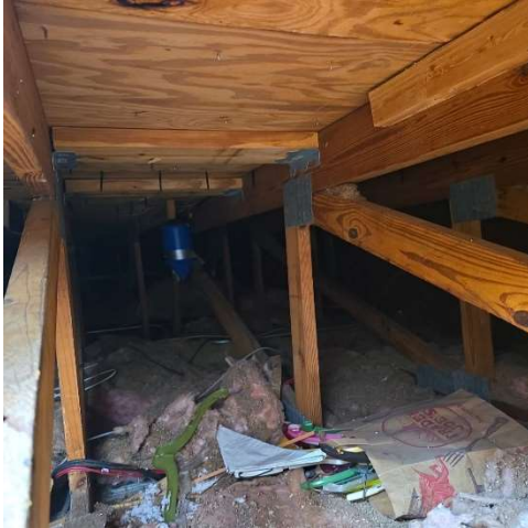
PHOTO-07 Roof Structure
