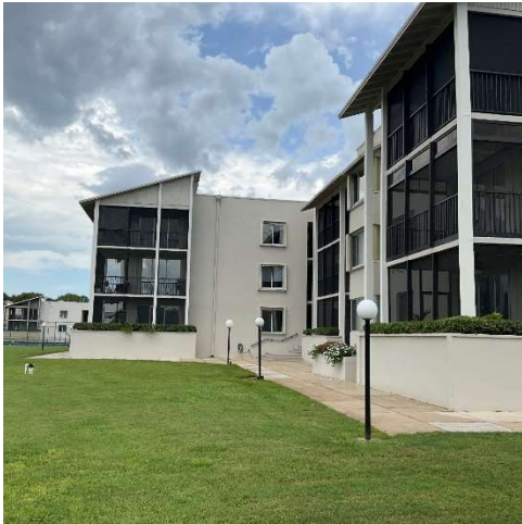
PHOTO-03 Building Exterior
